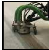
CURING COMPOUND REMOVAL
